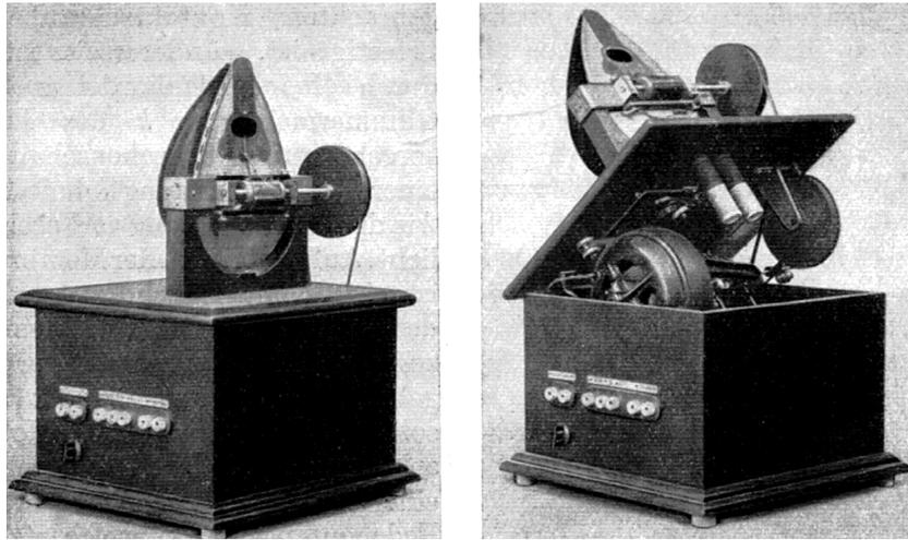
Figure 3.3: Example of a Johnson-Rahbek loudspeaker
